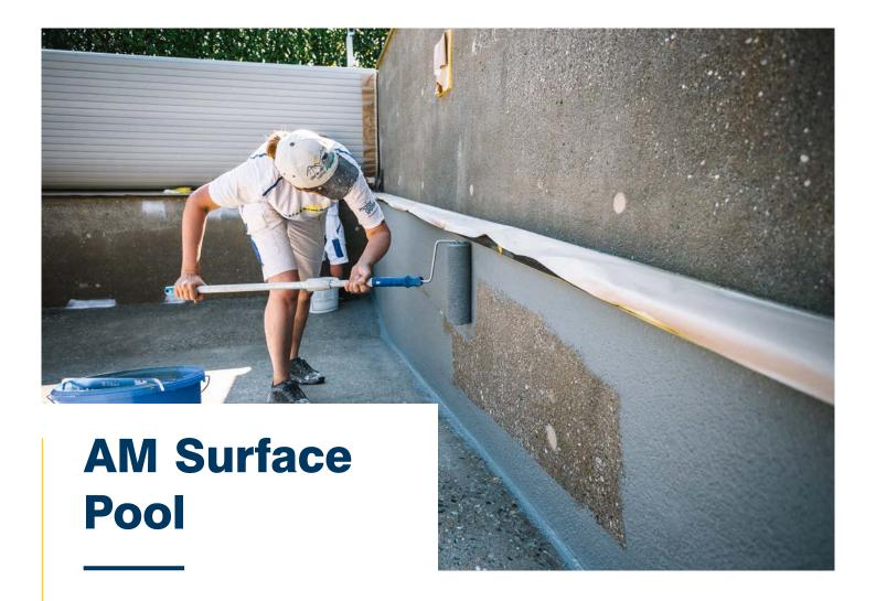
Dual-component protective coating based on polysiloxane epoxy resin.
